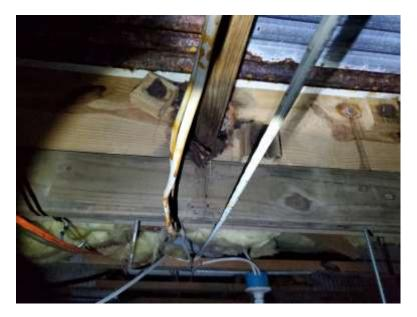
4. Oak Building: The railing along the back middle stair (south side) is corroded and needs supplemental reinforcement at 3 rail bases and at the bottom return.
