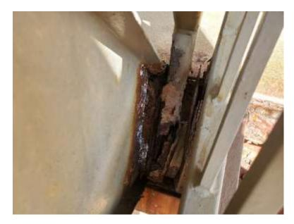
19. Willow Building: The railing along the back east stair (north side) has deteriorated at the rail bases and along the top rail, railing should be reinforced, and there are 2 loose steps that need to be re-anchored down.
