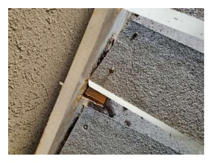
20. Willow Building: The steps along the back east stair (north side) have been removed. This stair should not be used unless NKU plans to reinstall the steps. THP review the front east stairs (south side), these stairs may be used at limited capacity as they were previously closed and not reinforced (second Photo).
