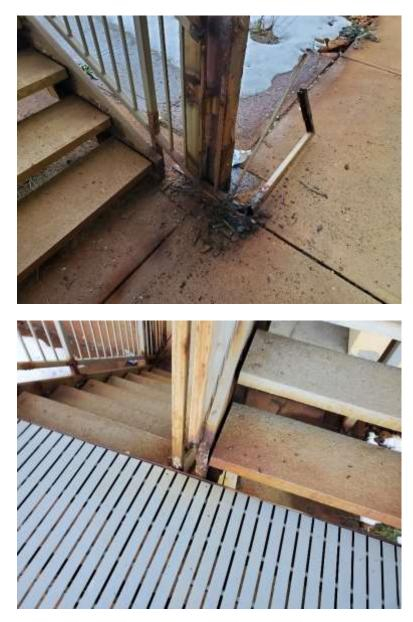
18. Willow Building: The railing along the middle front stair (south side) has deteriorated at multiple rail bases, and along the top of the railing. Reinforce railing at rail base.
