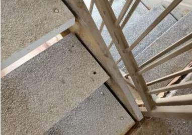
10. Sycamore Building: The railing along the back middle stair (west side) has deteriorated at the rail bases and along the top rail, railing should be reinforced, and there is 1 loose step that need to be re-anchored down.
