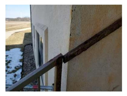
14. Sycamore Building: The remaining metal pan landings have further progressed in deterioration. No additional concrete spalls or missing pieces of concrete were noted. Photo is from the back (west side) south stair.
