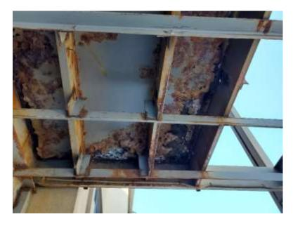
17. Willow Building: The railing along the middle back stair (north side) has deteriorated at each rail return, at multiple rail bases, and along the top of the railing. Reinforce railing at rail base and at rail returns.
