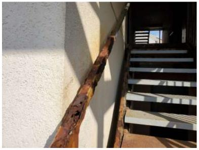
6. Oak Building: A railing along the back east stair (south side) is corroded and needs supplemental reinforcement.
