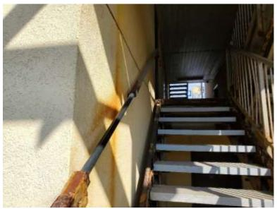
7. Oak Building: The railing along the front middle stair (north side) is corroded and needs supplemental reinforcement.
