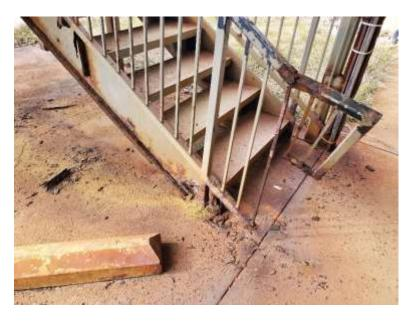
5. Oak Building: A railing along the back west stair (south side) is corroded and needs supplemental reinforcement.
