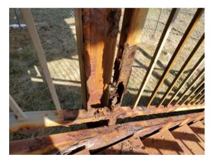
12. Sycamore Building: The front middle stair (east side) channel connecting the balcony walkway to the column is severely deteriorated with a 3Lf hole in the column. The connection to the previously installed reinforcing column is deteriorated and should be reinforced.
