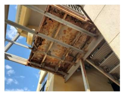
9. Sycamore Building: The railing along the south back stair (west side) has deteriorated at the rail base and along the top rail, railing should be reinforced, and there are 2 loose steps that need to be re-anchored down.
