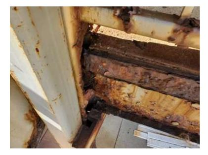
13. Sycamore Building: The railing along the north back stair (west side) has deteriorated split at the vertical post connection. Reinforce railing at rail base and to reconnected railing pieces.
