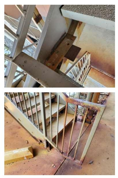
11. Sycamore Building: The railing along the front middle stair (east side) has deteriorated severely along the first run of stairs with the rail returns broken off, multiple holes in the top and bottom railing, and deteriorated rail bases. Railing should be reinforced.
