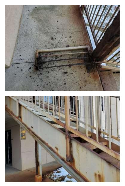
8. Oak Building: The remaining metal pan landings have further progressed in deterioration. No additional concrete spalls or missing pieces of concrete were noted. Photo is from the back (south side) east stair.
